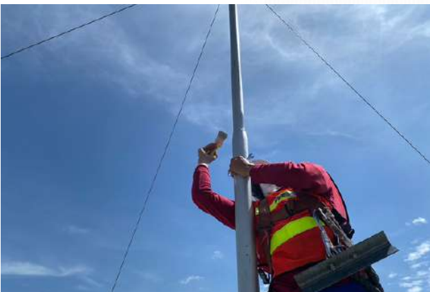
Mast Galvanized Steel Painting
