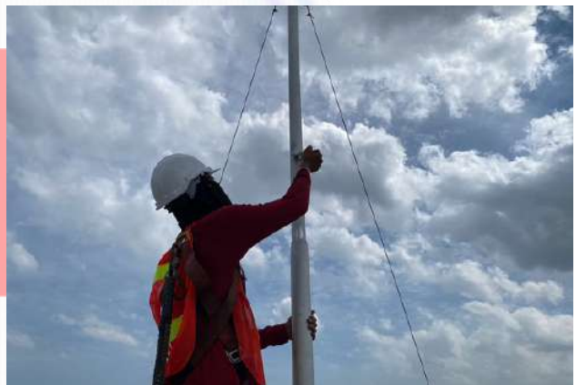
Mast Galvanized Steel Painting
