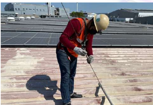
Lightning protection's sling checking
