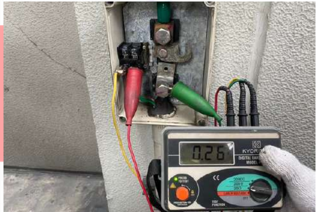
Test grounding resistance
