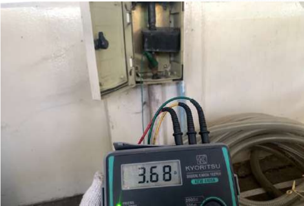
Test grounding resistance
