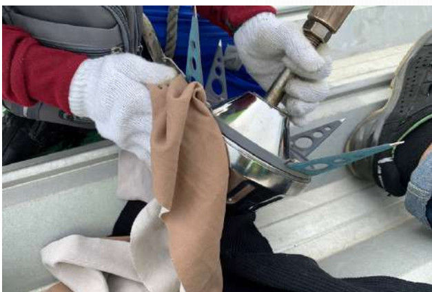
Head lightning protection cleaning
