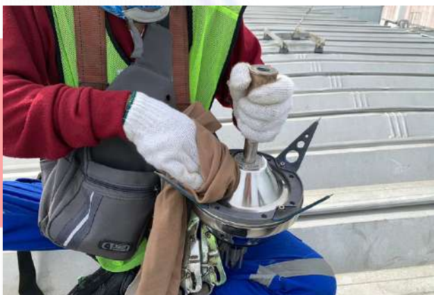
Head lightning protection cleaning
