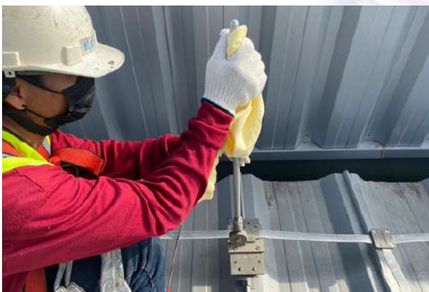
Lightning air terminal cleaning
