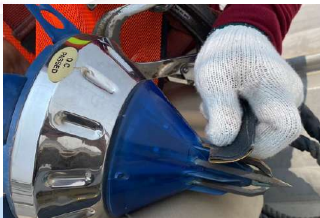
Head lightning protection cleaning
