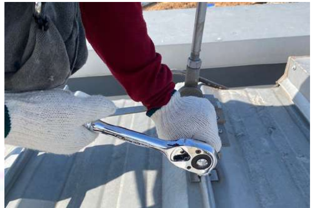
Check the degree of the lightning air terminal
